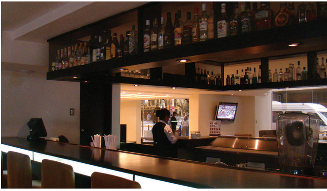
UniFi Access Point installed in hotel lounge
